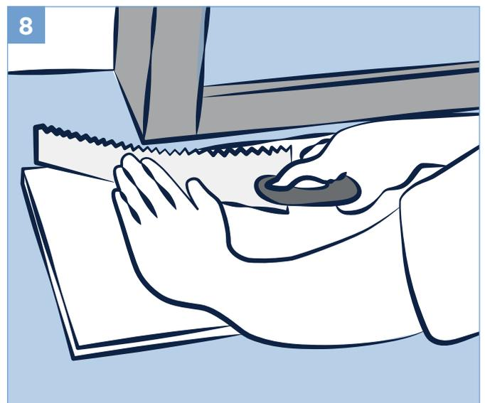
You can trim door frames by turning a plank upside down and using a handsaw to cut away the necessary height so that planks slide easily under the frames.
